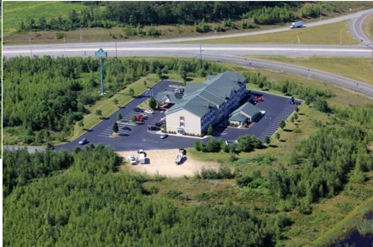
Country Inn & Suites Highridge Business Park Cass Township Schuylkill County Construction Completed — 2002 Jobs Created — 20
