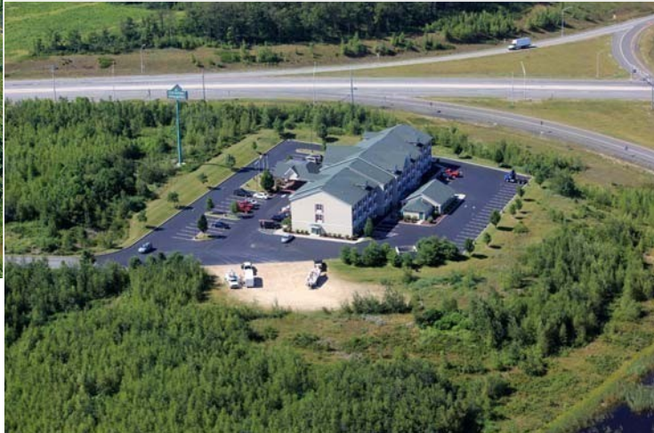
Country Inn & Suites Highridge Business Park Cass Township Schuylkill County Construction Completed — 2002 Jobs Created — 20
